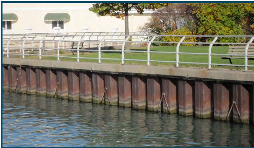
Steel Sheet Pile Wall East of St. Paul Pump Station (between Eastlawn Avenue and Lauzon Road)
