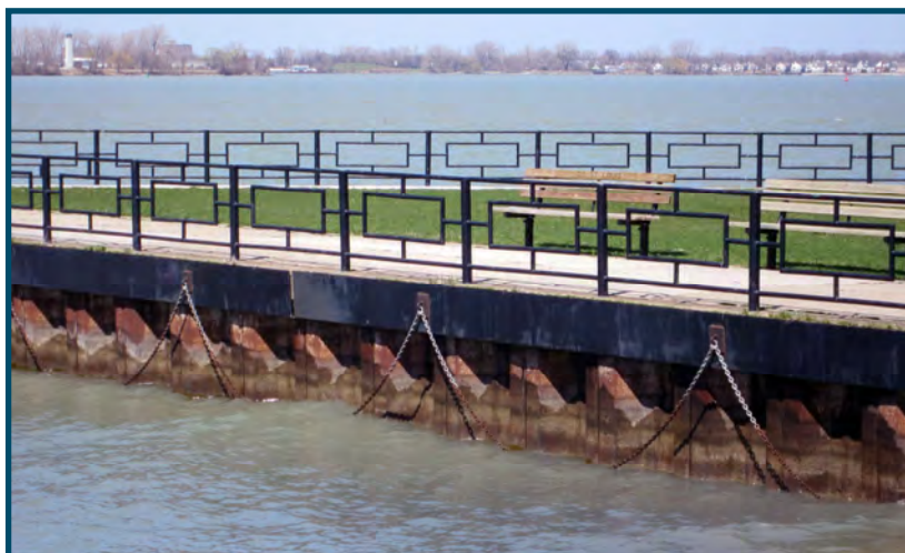
Steel Sheet Pile Breakwall at St. Rose Beach (at St. Rose Avenue)
