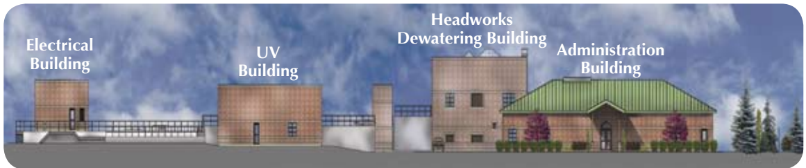
Overall facility as viewed from Sandwich Street
